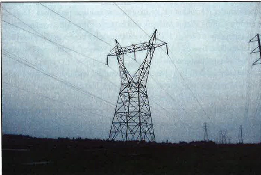
Figure 8. Historic Transmission Line, P-34-001102, view toward south
